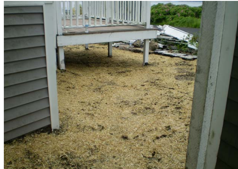
16. Hay cover to control moisture and erosion, June 21, 2017.
