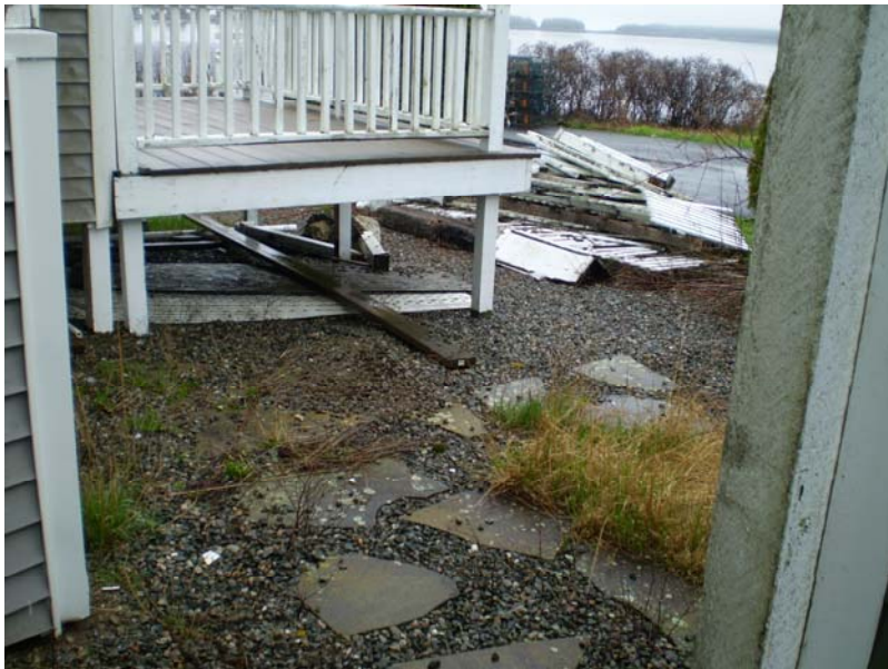
3. Site walk photo of soil removal area.
