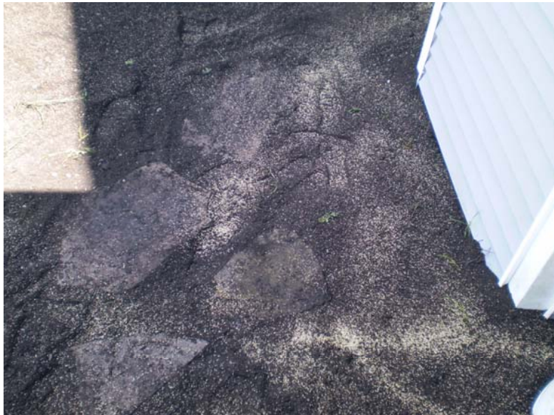
15. Topsoil seeded and pathway stones replaced, June 21, 2017.
