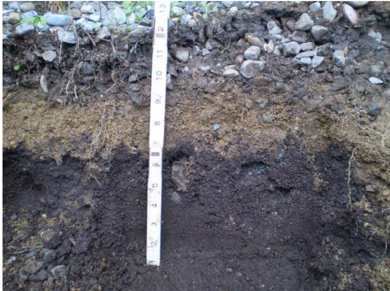
13. Soil was removed to a depth of 12 inches, June 20, 2017.
