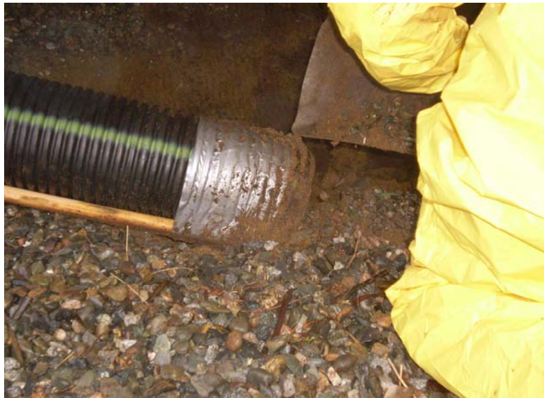
9. Soil removal by vacuum excavator, June 20, 2017.
