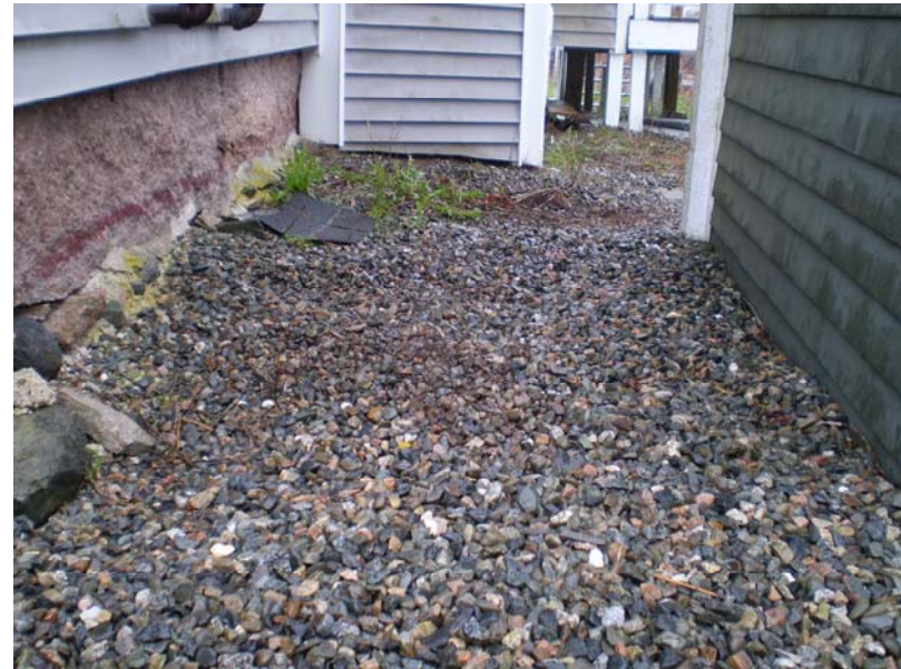
2. View south along western side of site building.
