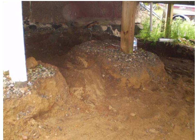
10. Area of excavated soil under deck, June 20, 2017.
