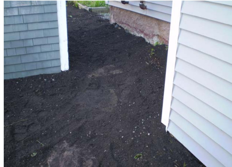
14. Area backfilled to original grade with clean topsoil, June 21, 2017.
