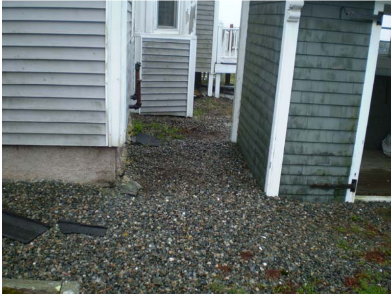
1. View south along western side of site building.
