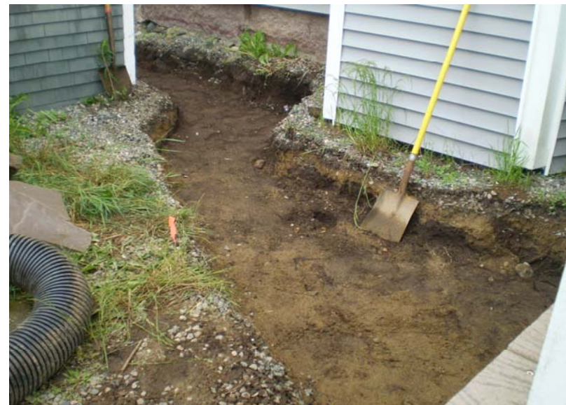
12. Area of excavated soil, June 20, 2017.
