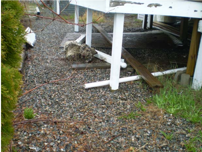
5. Site walk photo of soil removal area.
