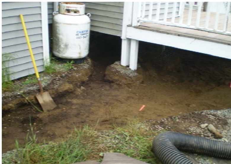
11. Area of excavated soil, June 20, 2017.
