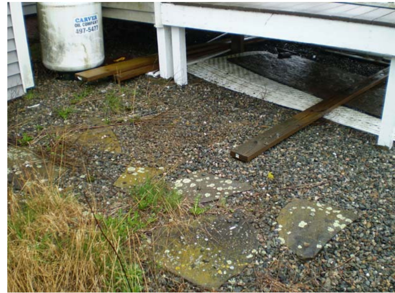
4. Site walk photo of soil removal area.
