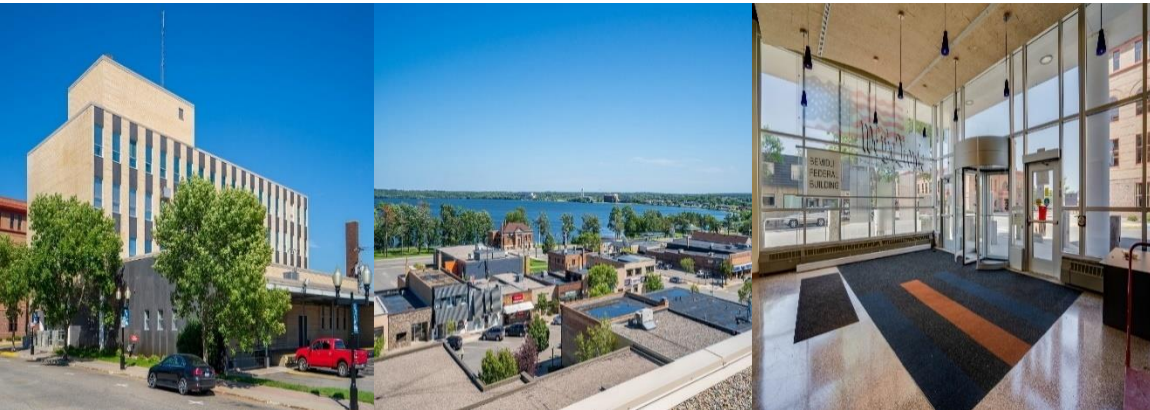
522 Minnesota Avenue North West Building (left to right): Entrance/Parking Lot, Rooftop, and Lobby area.
