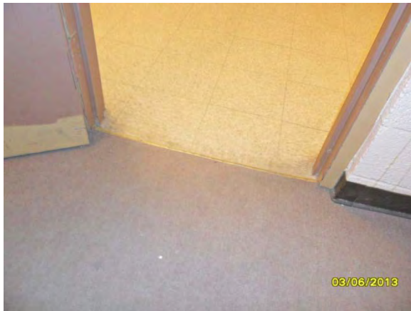
A-15. Administration Building, Transition from Main Hallway 102 to Room 111.
