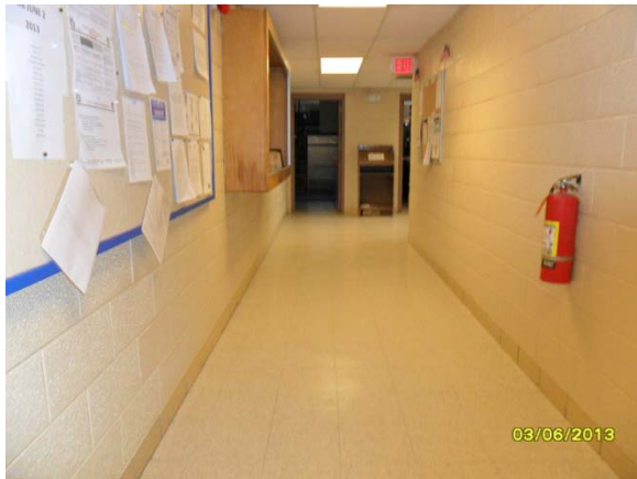
A-9. Administration Building, Hallway 102.
