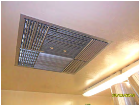
A-39. OMS, Break Room Ceiling.
