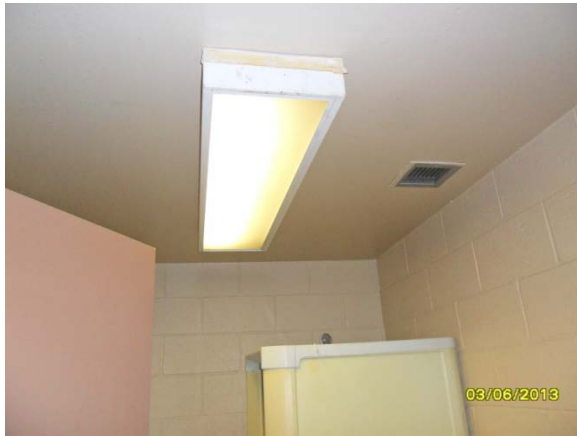
A-43. OMS, Break Room Latrine.
