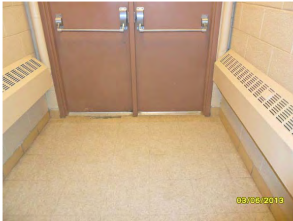
A-21. Administration Building, Main Hallway 102, West Exit.
