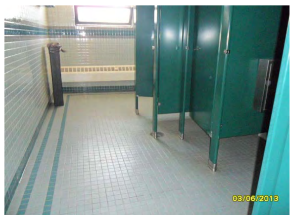
A-12. Administration Building, Women's Latrine, Room 107.
