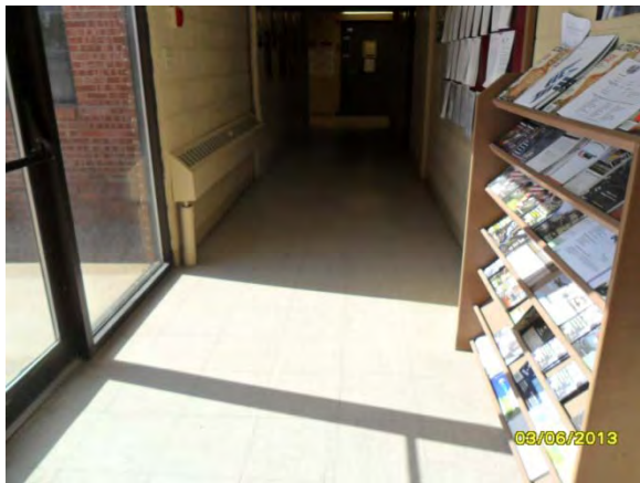
A-29. Administration Building, Hallway 103, Near East Entrance.
