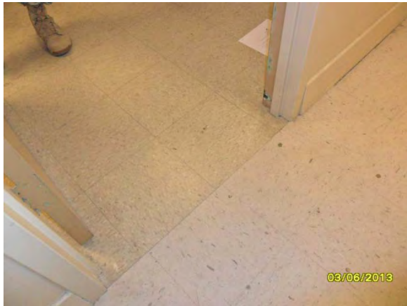
A-27. Administration Building, Hallway 103 and Room 119.
