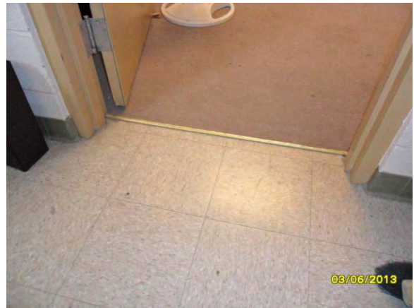
A-16. Administration Building, Transition from Main Hallway 102 to Room 112.
