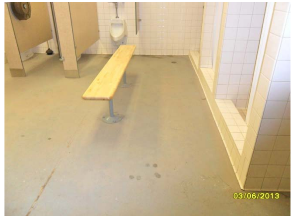
A-10. Administration Building, Men's Latrine, Room 116.
