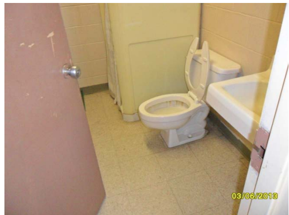
A-42. OMS, Break Room Latrine.
