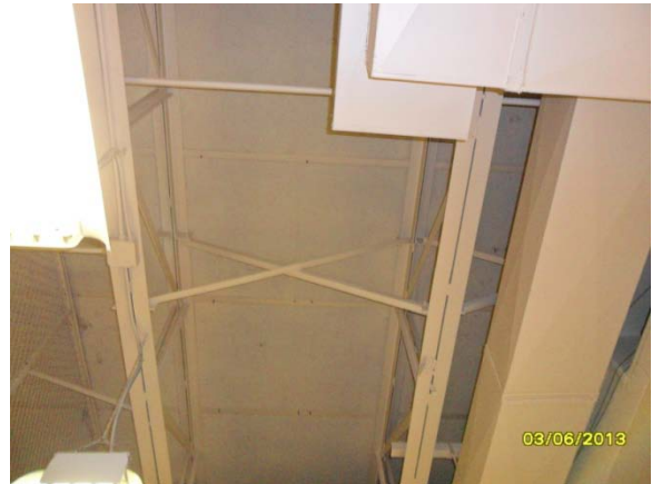
A-48. OMS, Service Area Ceiling.
