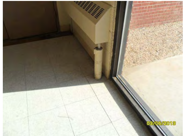
A-28. Administration Building, Hallway 103, Near East Entrance.
