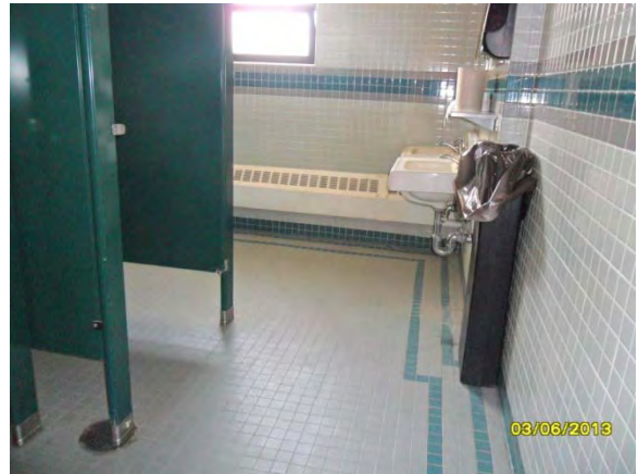
A-14. Administration Building, Women's Latrine, Room 107.
