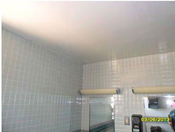
A-13. Administration Building, Women's Latrine, Room 107.
