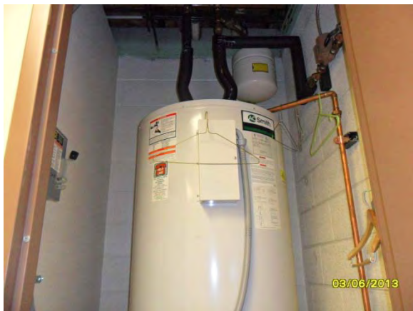
A-11. Administration Building, Men's Latrine, Utility Closet, Room 116.
