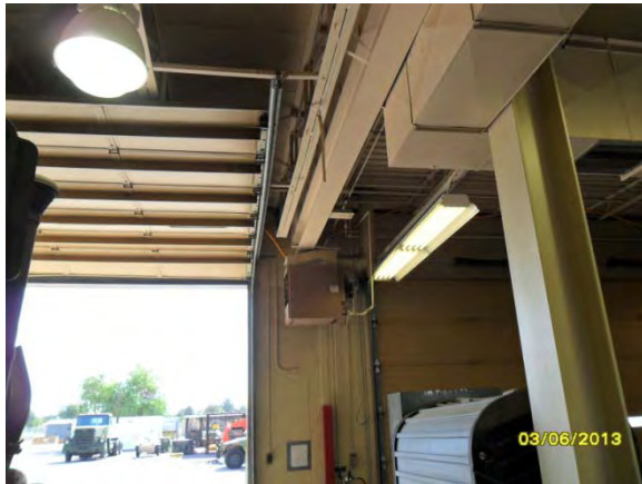
A-53. OMS Shop, Maintenance Bay Area.
