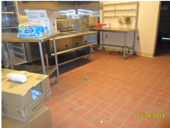
A-37. Administration Building, Kitchen, Room 120B.
