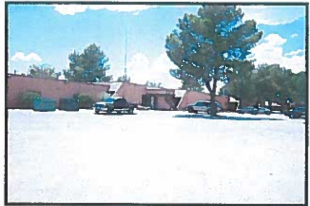
View of subject site looking southwest from east end
