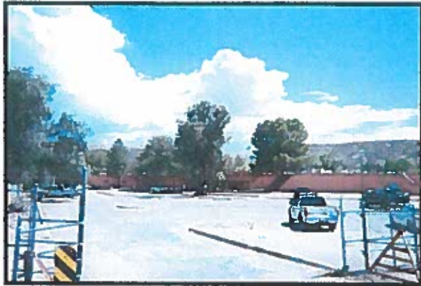
View of subject site looking south from Highway 170
