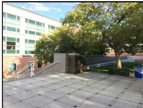
Overall – Source Pool, Stream Bed, Runnel, Backrest Screen and Vortex
